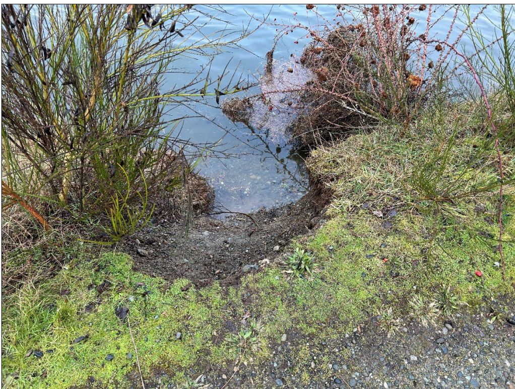
Example of erosion on Dike 49
