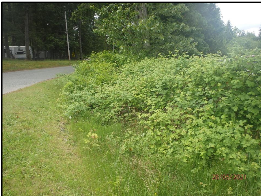
Looking upstream at the section of ditch that runs along Chapman Road, west of the property entrance. As can be seen in the photo the channel is fully overgrown with grasses and Himalayan blackberry.
