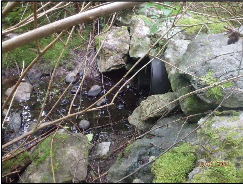
A photo of the culvert that conveys water from the outlet drainage subsurface. From this point the flow of water is entirely underground until it reaches the roadside ditch adjacent to Chapman Road.
