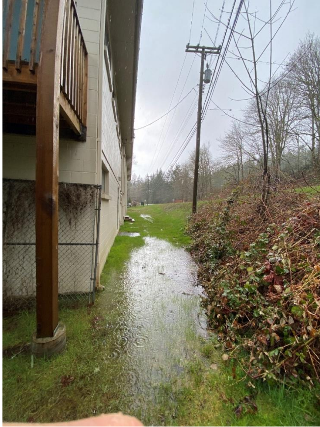
Figure 5: Ponding during rain event North of Gymnasium adjacent Shawnigan Lake Road that has no formal roadside ditch along this length of the road
