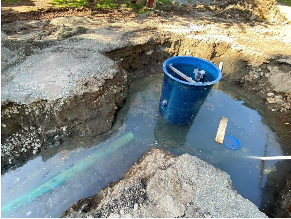
Figure 7: View of excavation in camp area showing shallow water table.
