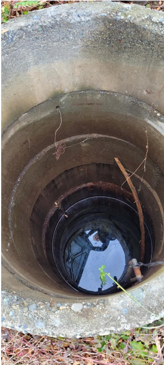
PHOTO 10. VIEW LOOKING DOWN A GROUNDWATER WELL LOCATED PROXIMAL TO THE FORMER RESIDENCE. STATIC WATER LEVEL DURING THE TIME OF MADRONE'S ASSESSMENT WAS ESTIMATED TO BE ~ 1.5 M. PHOTO DATED FEBRUARY 22, 2023.
