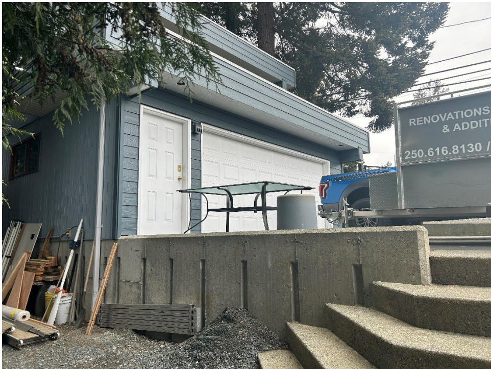
April 12, 2024 – Retaining wall on north side of driveway, to be used as foundation for proposed carport
