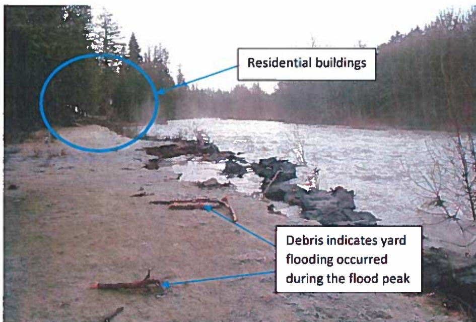
Photo 1: Example of private property flooding on 1 February 2020. Yard areas were flooded but water levels reached few buildings. Riprap revetments were overtopped, resulting in bank washout
